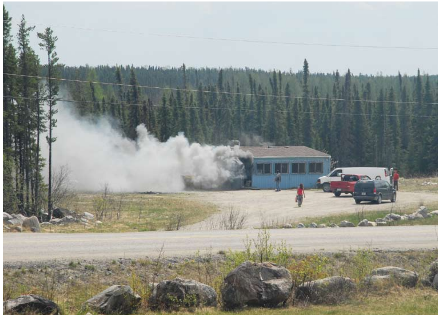
Fire destroyed the old finance building which had been converted to a thrift store and was to become a youth centre at Ten Houses.
